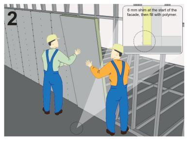
With the help of a partner, place the panel in the desired location. At the start of the façade, leave a gap of 6 mm using the grey shims, position and level the panel. These 6 mm will be filled with TABIHAUS® polymer.
