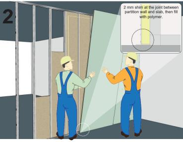
With the help of a colleague, place the panel in the desired location. Place a 2 mm shim at the joint between the partition wall and the floor slab, then fill with polymer.
